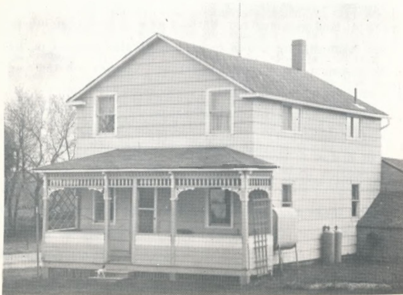
The above building on the northwest corner of Lower Ratho, at present the home of Mr. and Mrs. James Pettigrew, was formerly owned by Nicholas Smith and operated as a Wagon Shop. It had a ramp on the front by which buggies and wagons could be taken to the second storey.
