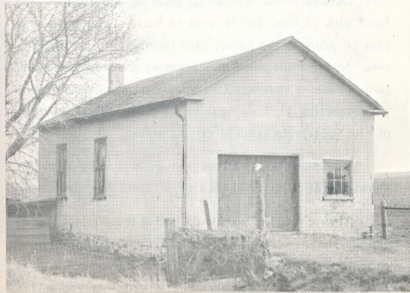
The above building is the Forester's Hall situated west of the corner at Lower Ratho on Concession 12. Until recently this hall was the centre for many and varied community activities.
